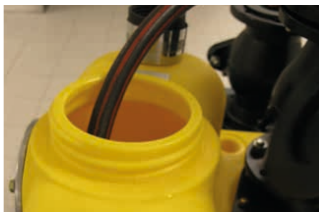
▶ Cleaning the tank
