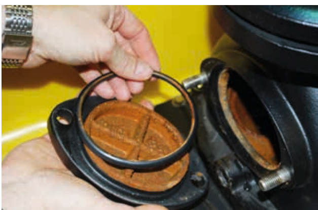
▶ Checking and cleaning the swing-type check valve
